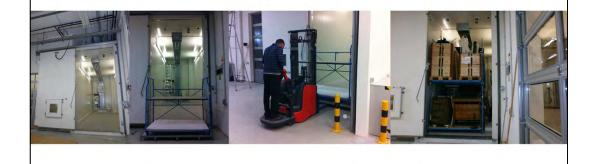
As part of pest control we have a new nitrogen chamber with a ground area of about 22m2 (7.5m length x 3m width x 4.5m height) and a capacity of about 100m3.
